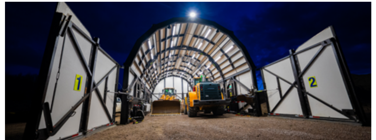
Work in a daylight environment thanks to the 28 interior LED fixtures (48W/5 000 lumens).
